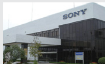
Sony Chemicals (Suzhou), site of the first BOO project for wastewater recycling
