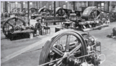
Part of the ammonia plant completed in 1923 (Nobeoka, Miyazaki, Japan)
