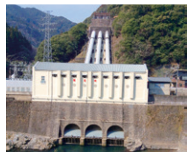
The Gokase River Hydroelectric Plant
