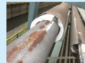
Example of CUI inspection by removing insulation
