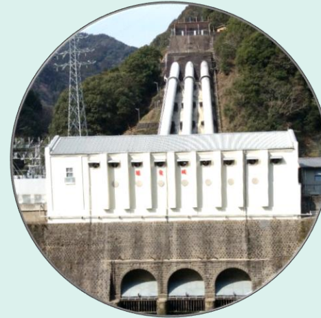
Hydroelectric power plant in Miyazaki, Japan
