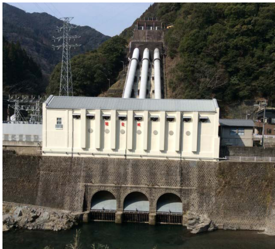
Gokasegawa power plant
