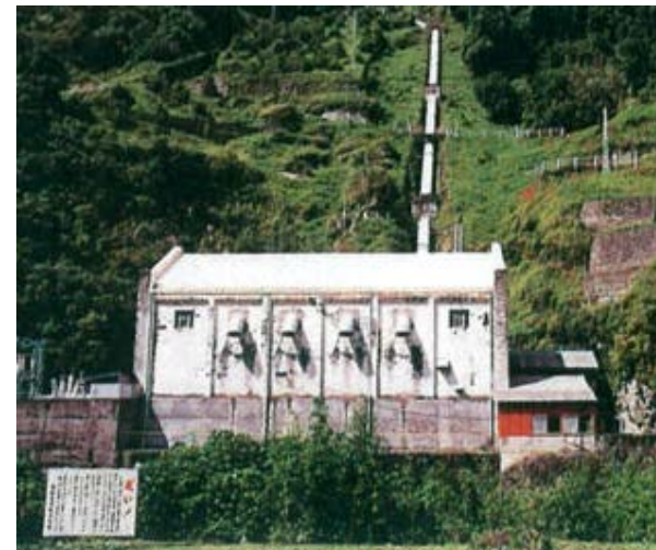
Mamihara power plant
