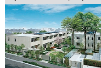
Hebel Maison™ apartment building
