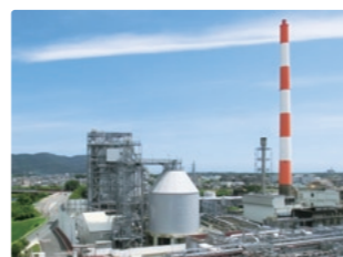
The new plant
