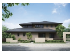
Two-story Hebel Haus™
