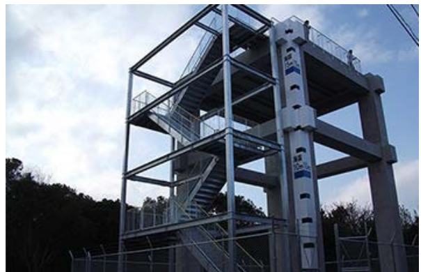
Evacuation tower in Nobeoka, Miyazaki Prefecture
