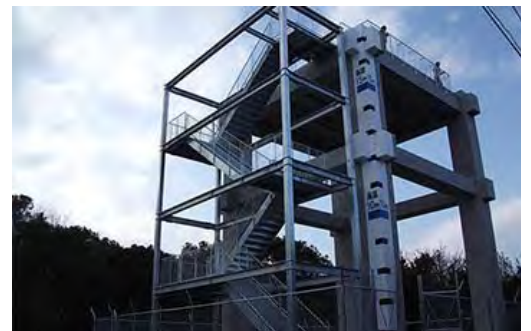
Evacuation tower in Nobeoka, Miyazaki Prefecture
