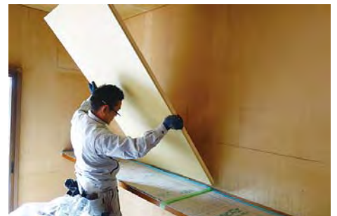
Retrofitting the insulation board on an existing wall
