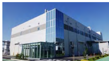
Asahi Kasei Fuji facility for commercial production of UVC LEDs
