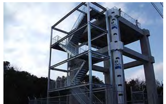
Evacuation tower in Nobeoka, Miyazaki Prefecture
