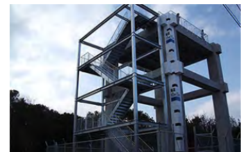
Evacuation tower in Nobeoka, Miyazaki Prefecture
