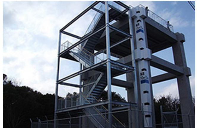
Evacuation tower in Nobeoka, Miyazaki Prefecture
